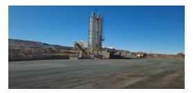
A concrete batch plant was commissioned in early 2018. The plant is capable of 80m<sup>3</sup> of general use concrete per hour. The plant will be used in the operational restart and construction phase for the concrete demand from these activities.
