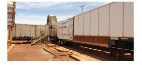
Nifty generates its own power from a gas fired captive General Electric 21MW power plant. Nifty also has on standby two 2.5MW gas / diesel turbine generator sets, two 2MW diesel generator sets and two 1MW diesel generator sets.
