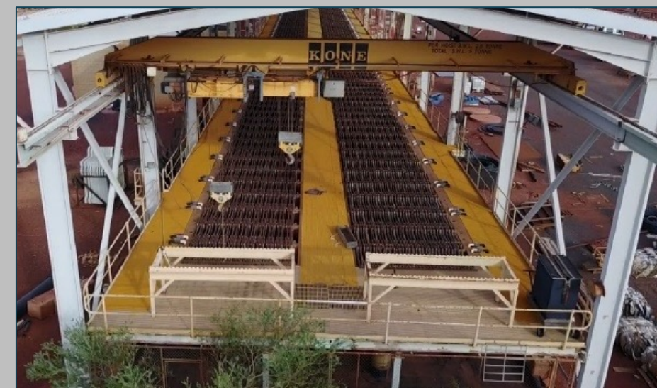
Brownfield Cathode Plant
