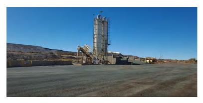
A concrete batch plant was commissioned in early 2018. The plant is capable of 80m<sup>3</sup> of general use concrete per hour. The plant will be used in the operational restart and construction phase for the concrete demand from these activities.
