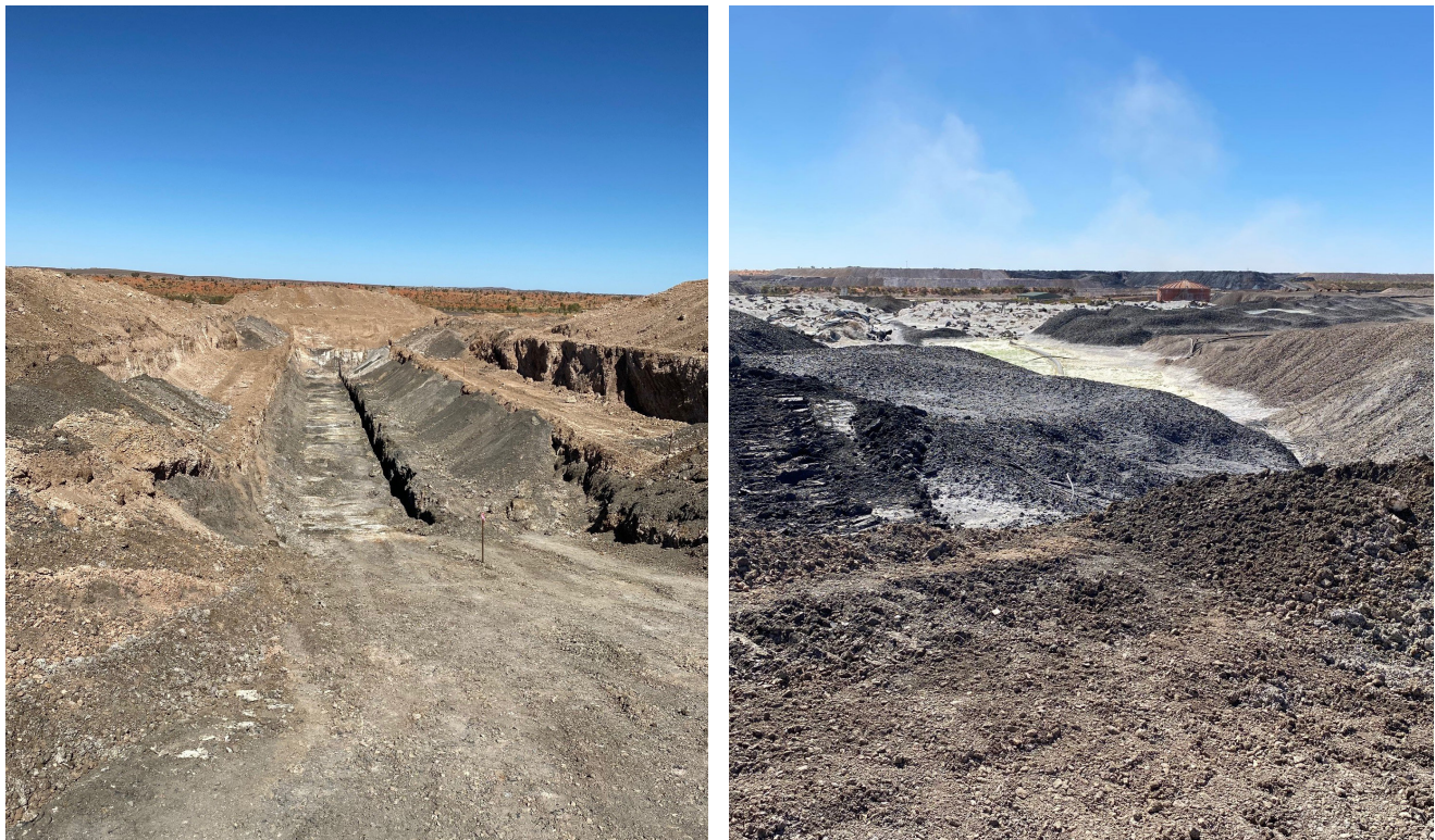
Fig 3. Nifty – Heap Leach Trenching (LHS) and Old Pad (RHS)
